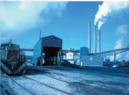
Feeders located beneath steel grating and storage hoppers at a rail car unloading station located outside Louisville, Kentucky.
